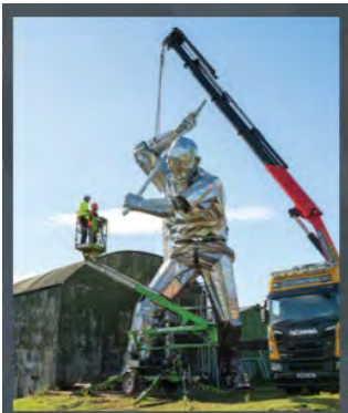
John McKenna at the test build. The figures were made in sections in the studio and assembled outdoors with the aid of cranes and elevators.
